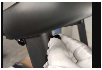
**Step 2:** locate the screw near the wheel either side. Unscrew this screw on both sides as shown below.
